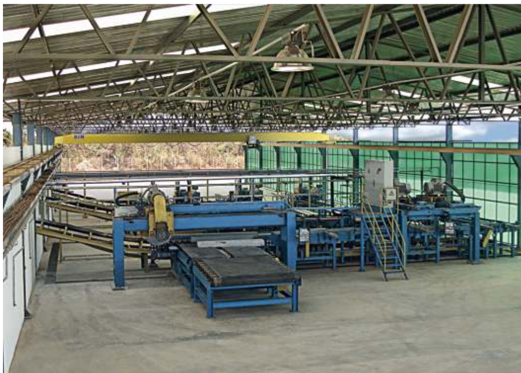
Roofing Slate Unit - the world's second largest automated roofing slate plant
